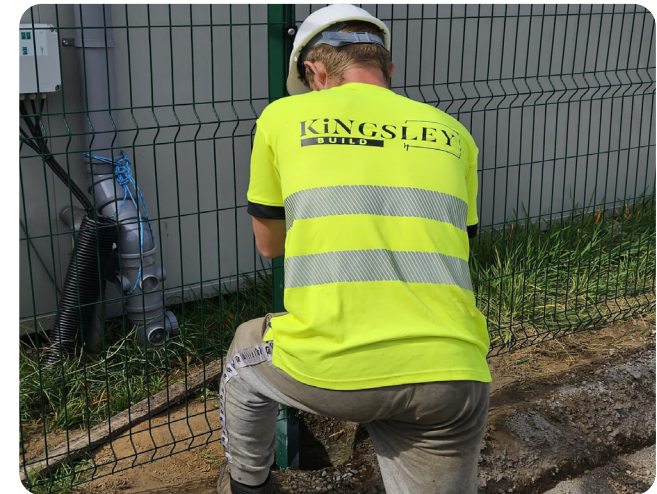
Kingsley Build School Fencing Project - Pre-installation Works
